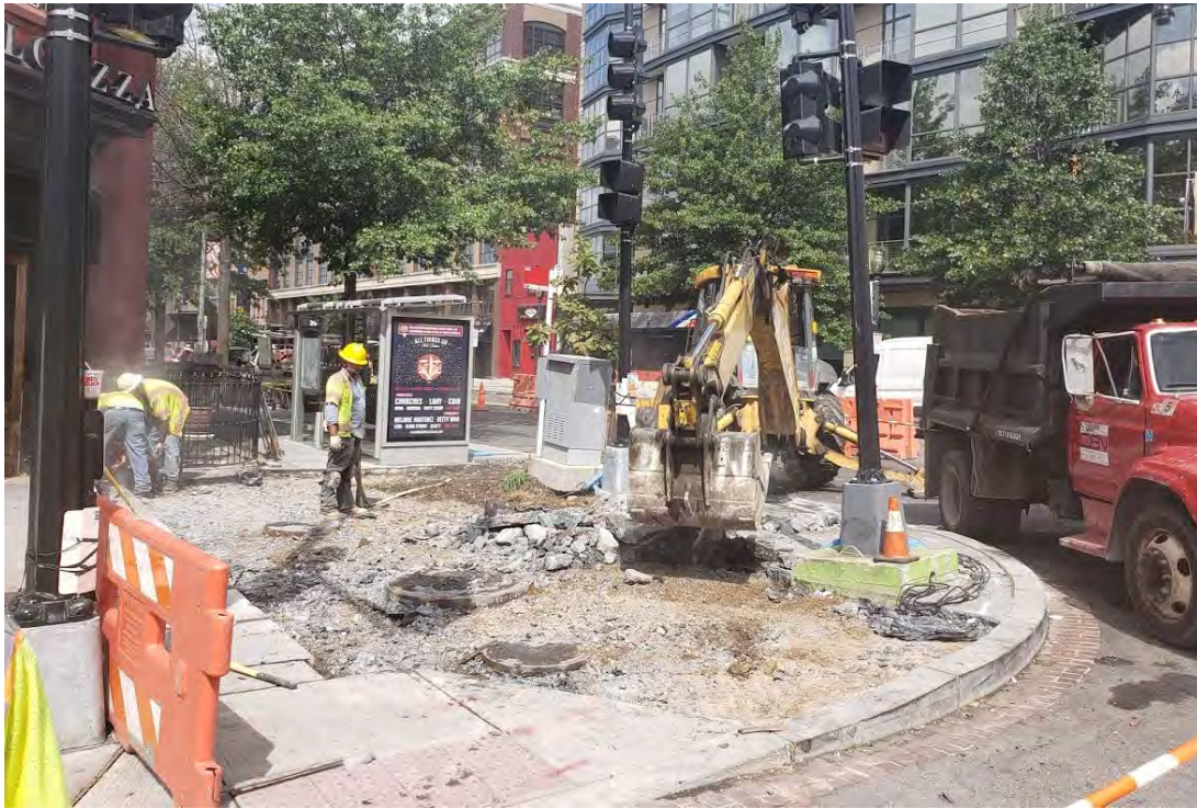
DEN excavating for sidewalk installation at 14 th St. & P Street
