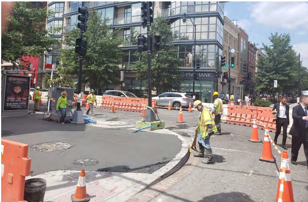
DEN completing sidewalk finish work at 14th St. & P Street
