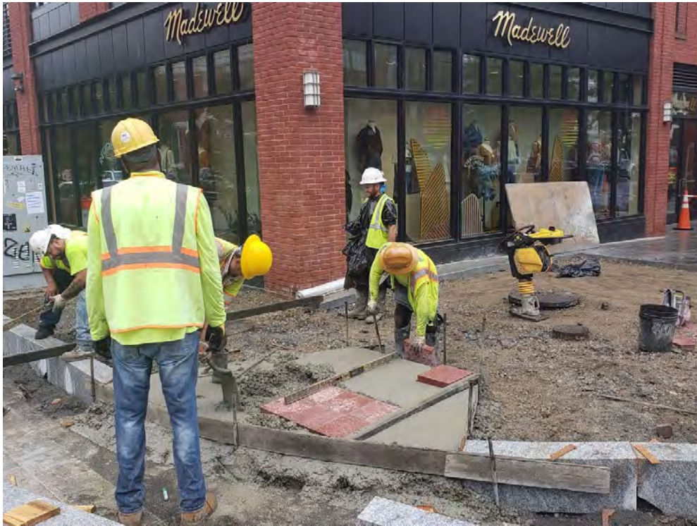
ADA ramp construction at 14 th St. & Wallach (NB)
