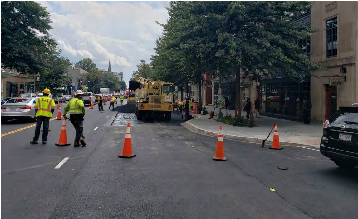
Paving parking lane going SB on 1500 block of 14 th St. NW
