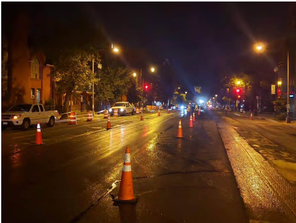
Proper MOT established along 14 th St. during night shift paving operations
