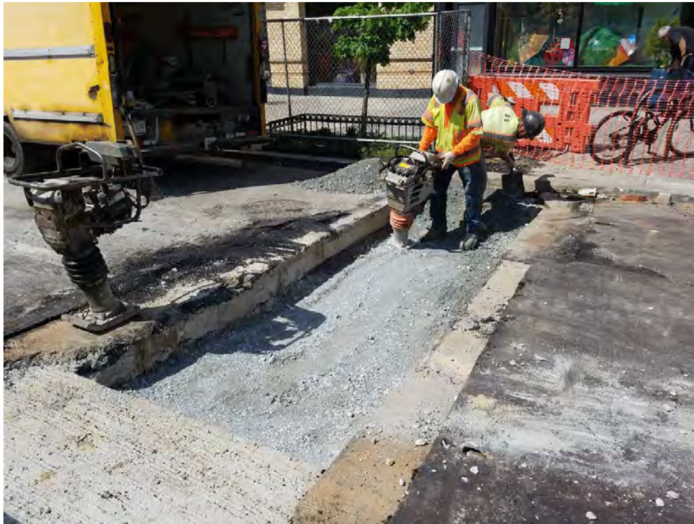
Compaction of Aggregate Base Material over Water Service Line
