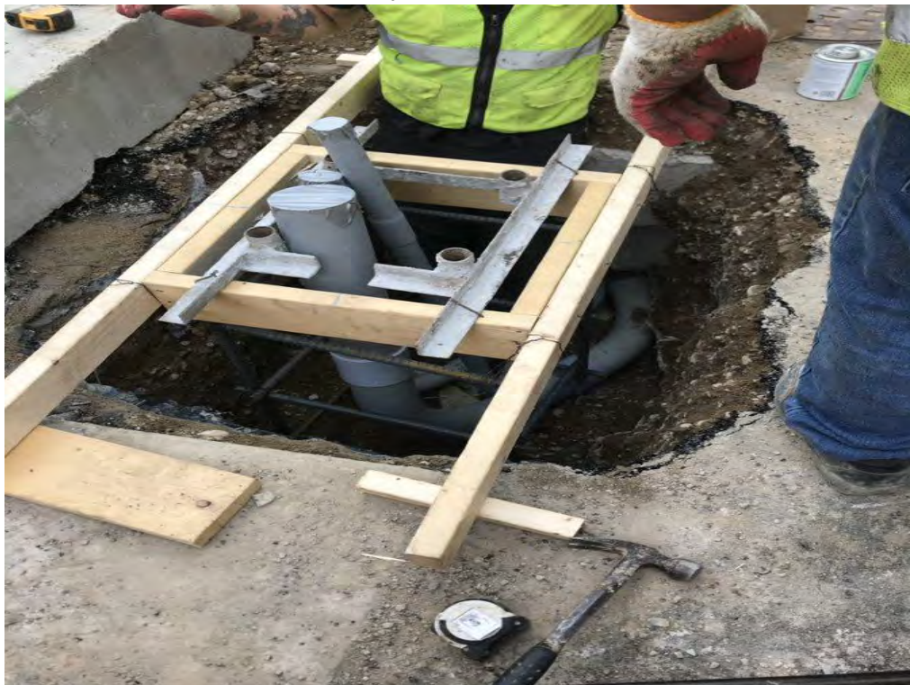
Installation of New Fire Hydrant between V Street and W Street
