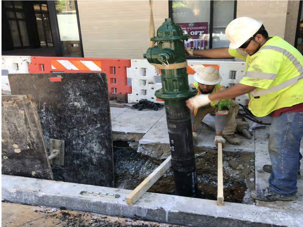
Installation of New Fire Hydrant between V Street and W Street
