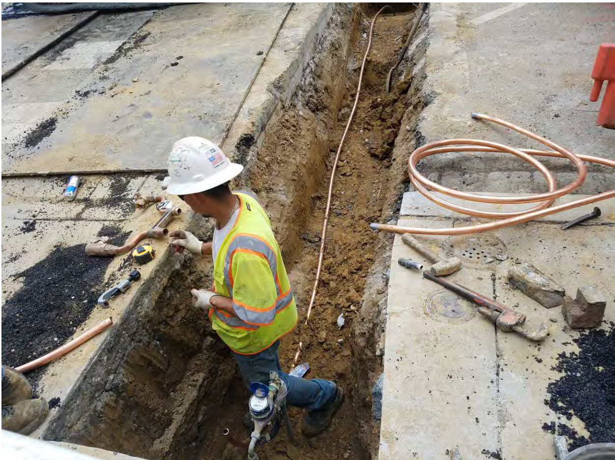
Installation of 2" Water Service Line between R Street and Street
