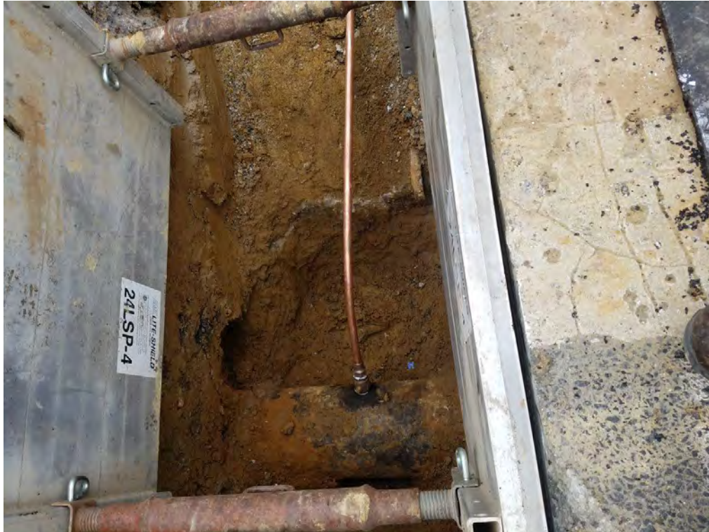
Insttation of New Water Service Line into 12" Watermain
