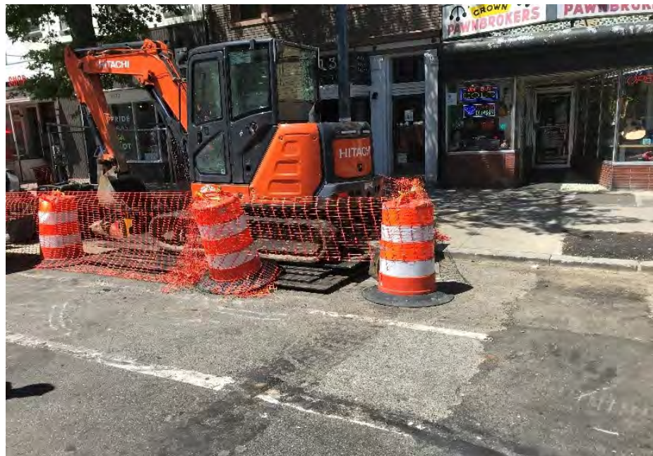
Contractor left the site safe and secured over the weekend.
