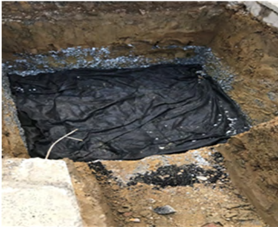
Installed #57, bedding stone and geotextile fabric for the electric manhole M52
