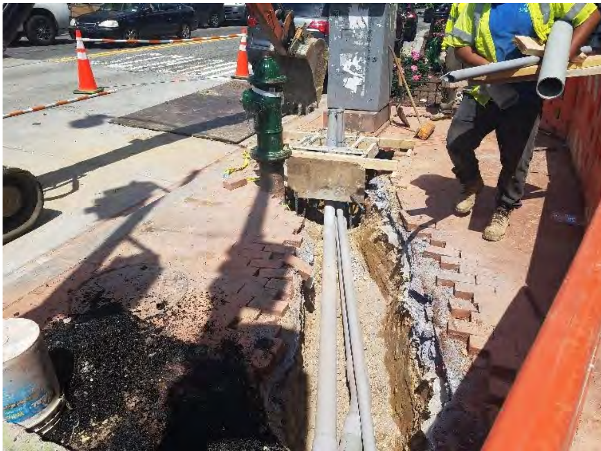
East view of M108 to TC-11 PVC trench
