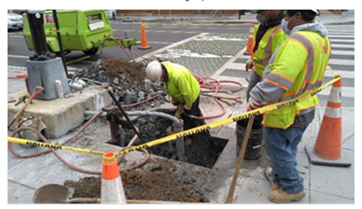
Demo and removal of cracked foundation Q Street
