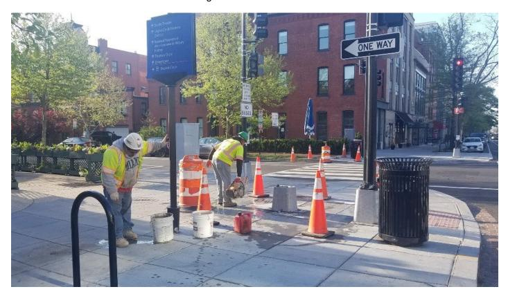
FMCC working on removing the T-base at NEC of Q Street
