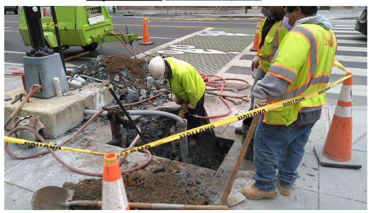
FMCC Restoring damaged Signal foundation at Q street
