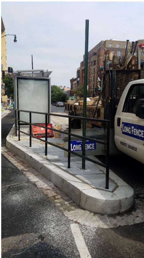
Long Fence installing handrail at the N street Bus Island
