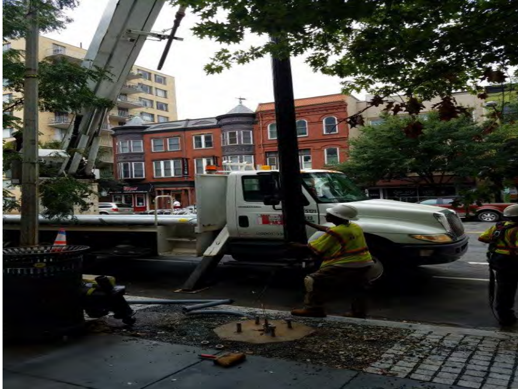
Installation of Twin 20 Street Light Pole
