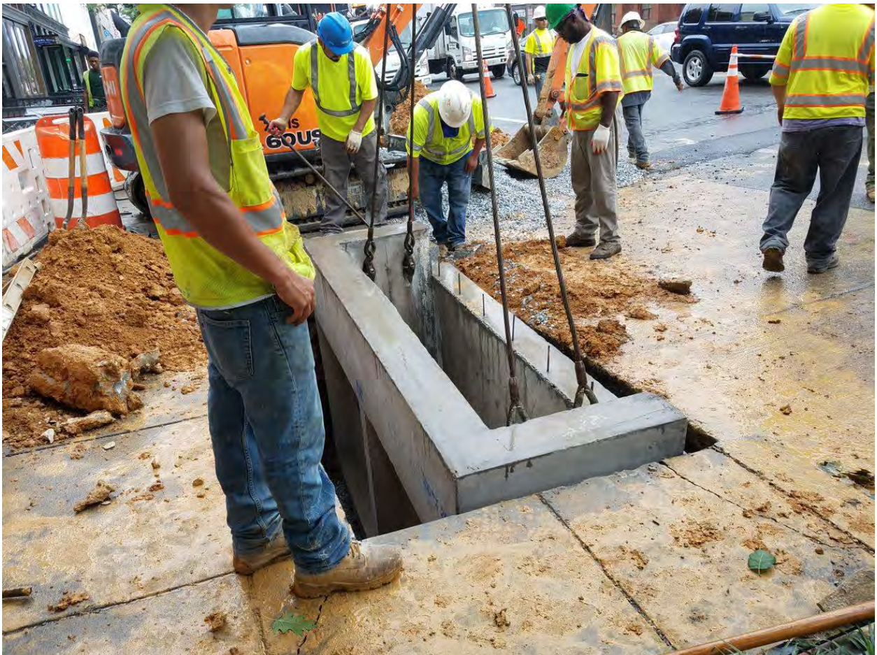
Installing the Double Catch Basin at between P and Q Street
