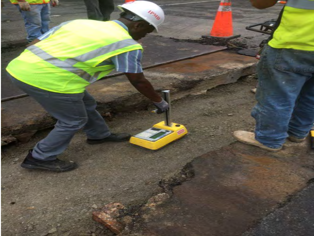
QA/ QC testing for compaction of Aggregate Base Material
