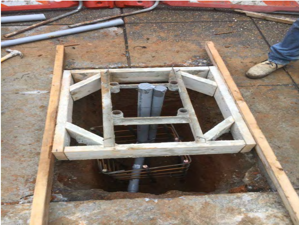
Form work for Street Light Foundation
