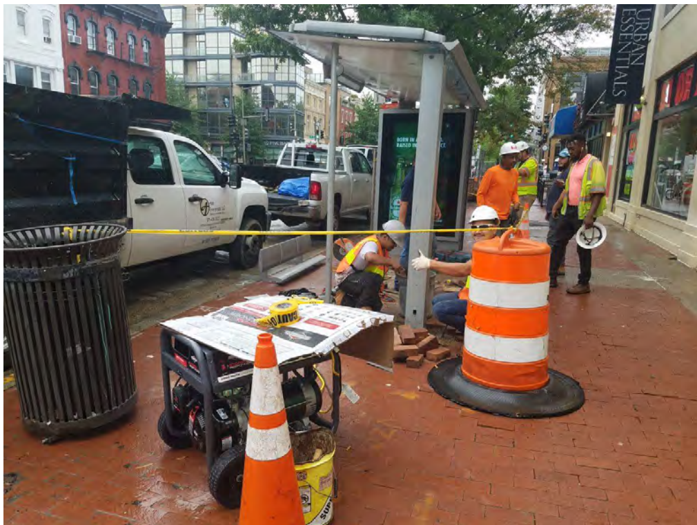
Clear Channel Removing Glass from Bus Shelter prior to removal
