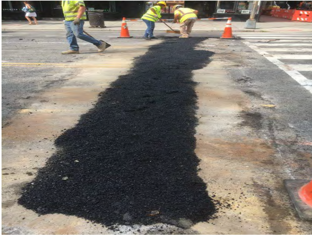
Placing Temporary Asphalt over PCC Base
