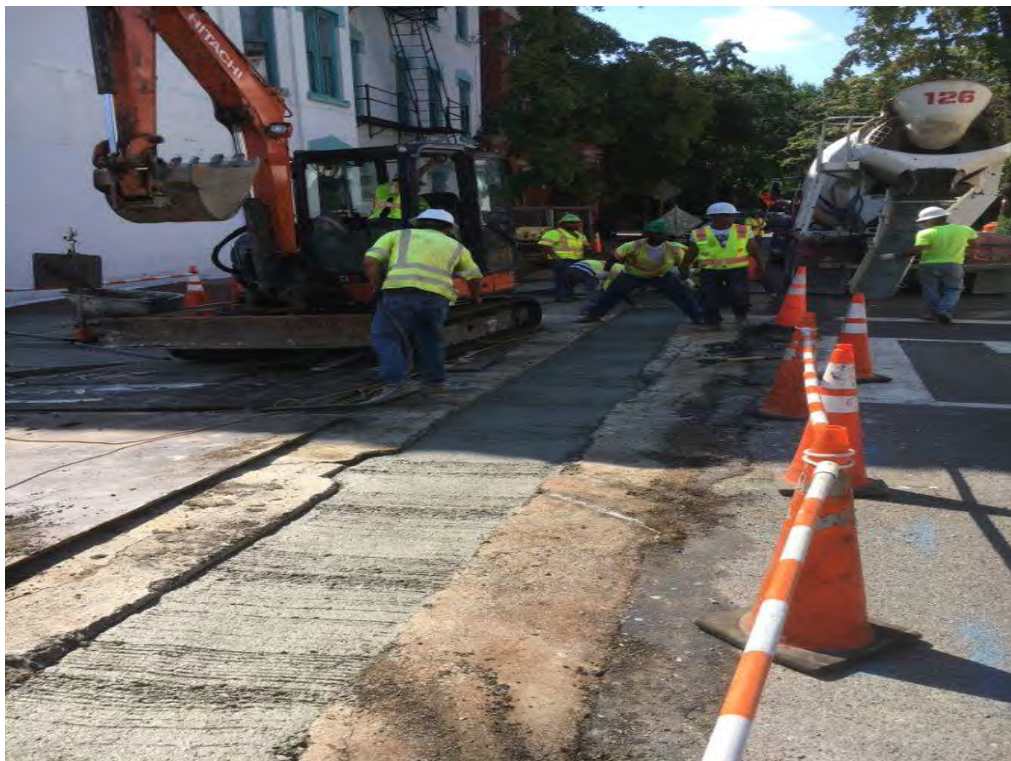
Placing PCC Base over PVC Conduit Trench
