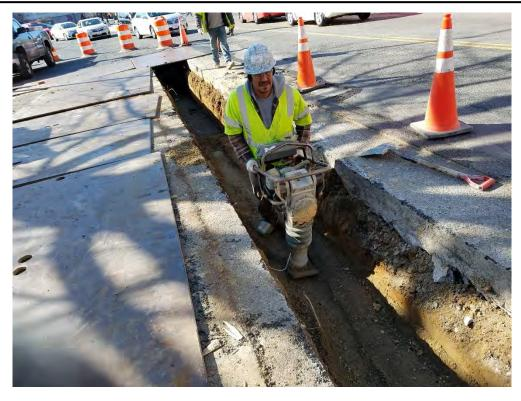
Compaction of Backfill Material over encased PVC Consuit
