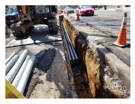
Installation of 6-4" and 1-2" PVC Conduit
