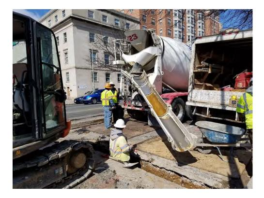
Placing PCC Concrete for encasement of PVC Conduit
