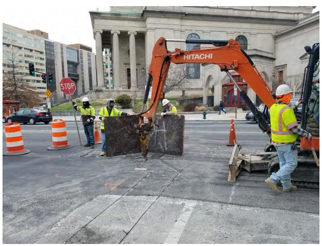
Demoliation of pavement for conduit installation between Thomas Circle and N Street on the Eastside
