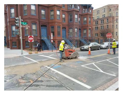
Saw-Cutting on N Street for Manhole installation
