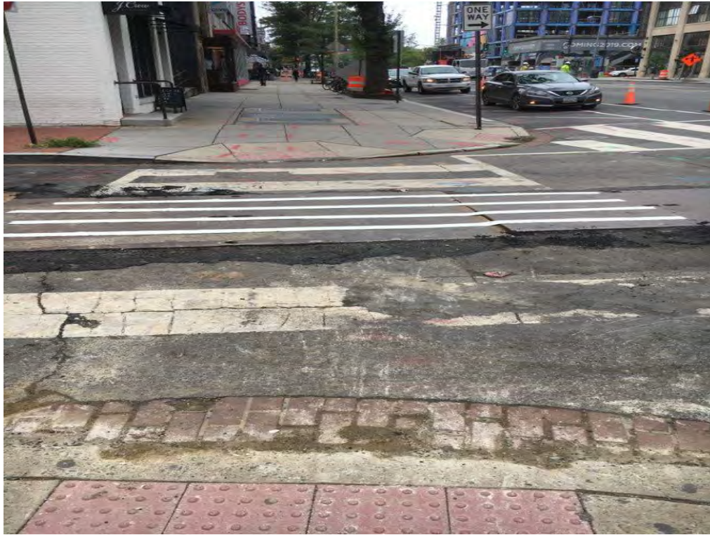
Safety strip placed over Steel Plate
