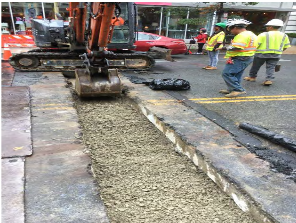
Scarfig Backfill Material to assist in drying of wet material
