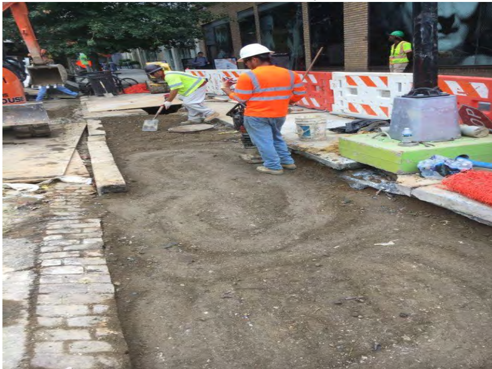
Backfilling of 15" PCC connection pipe for CB-07
