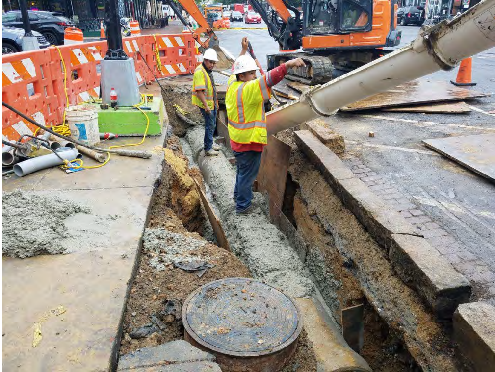
Pouring DC WASA mix for the PCC connection pipe cradle
