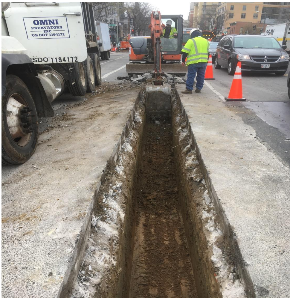
Excavation between Rhode Island Ave and P Street on the Eastside
