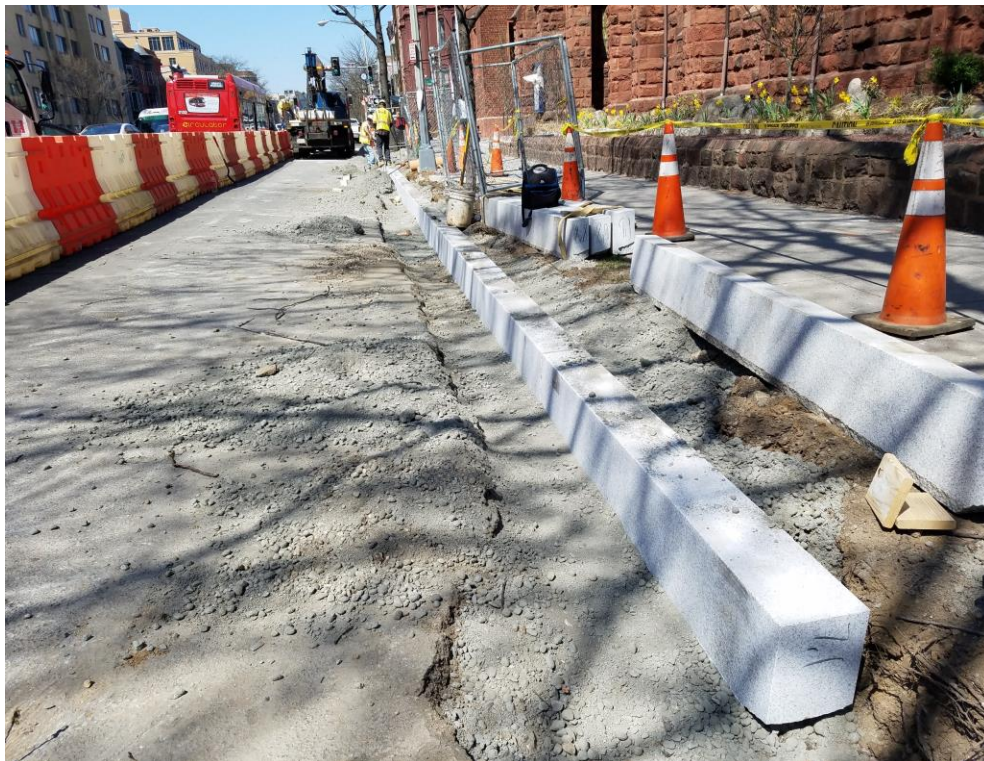
Placement of Granite Curb between Thomas Circle and N Street
