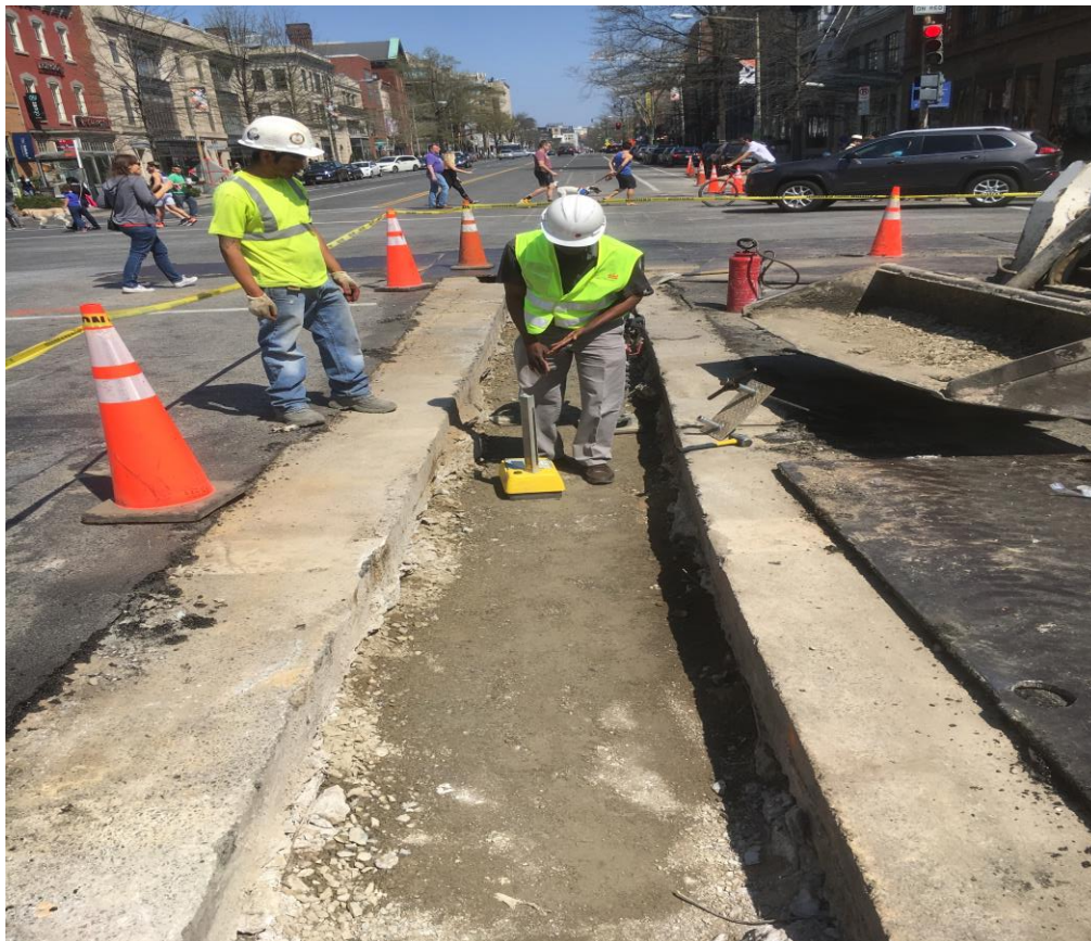
Compaction of Aggregate Base Material between Rhode Island and P Street
